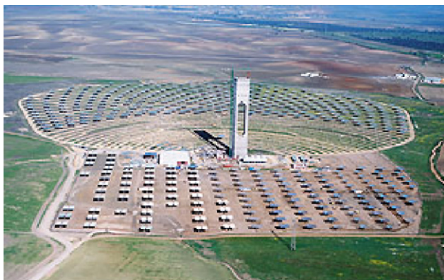
Fig. 4. Abengoa solar plants in Sanlúcar La Mayor [2].
